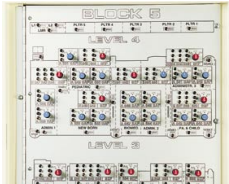
Fire Fan Control Panel 28U Typical MX4428 Rack 192 Zones maximum
